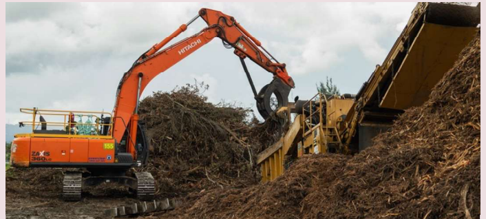
Mulching storm debris (January 2024)
