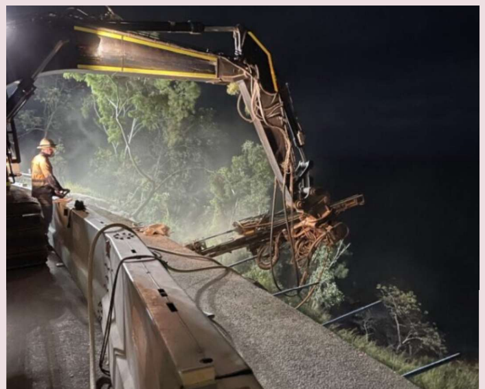
Critical slope stabilisation works (May 2024)
