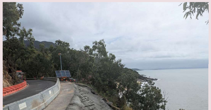
Completed critical slope stabilisation works (July 2024)
