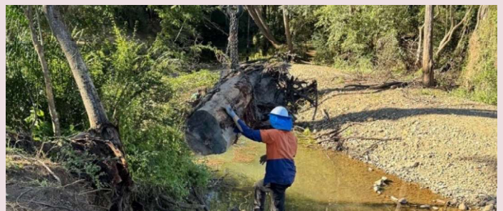
Tree root balls used in Cedar Creek stabilisation works
