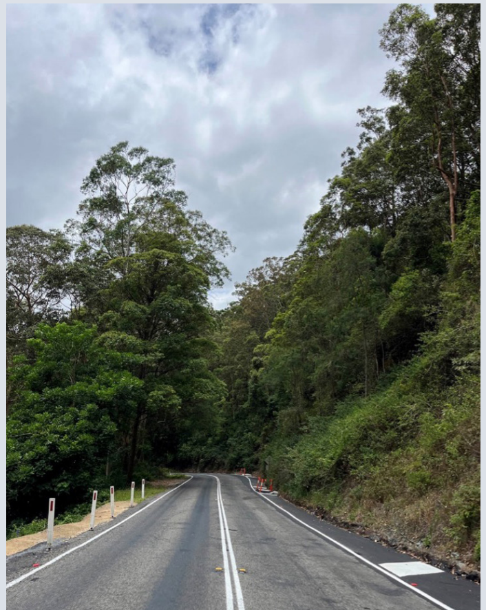
Pine Creek Road – completed emergency works
