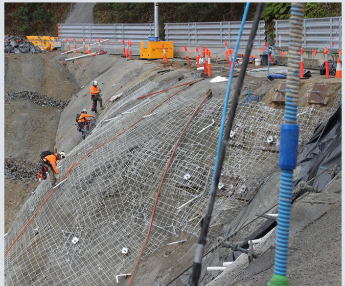
Beechmont Road – downslope stabilisation works in progress (December 2022)
