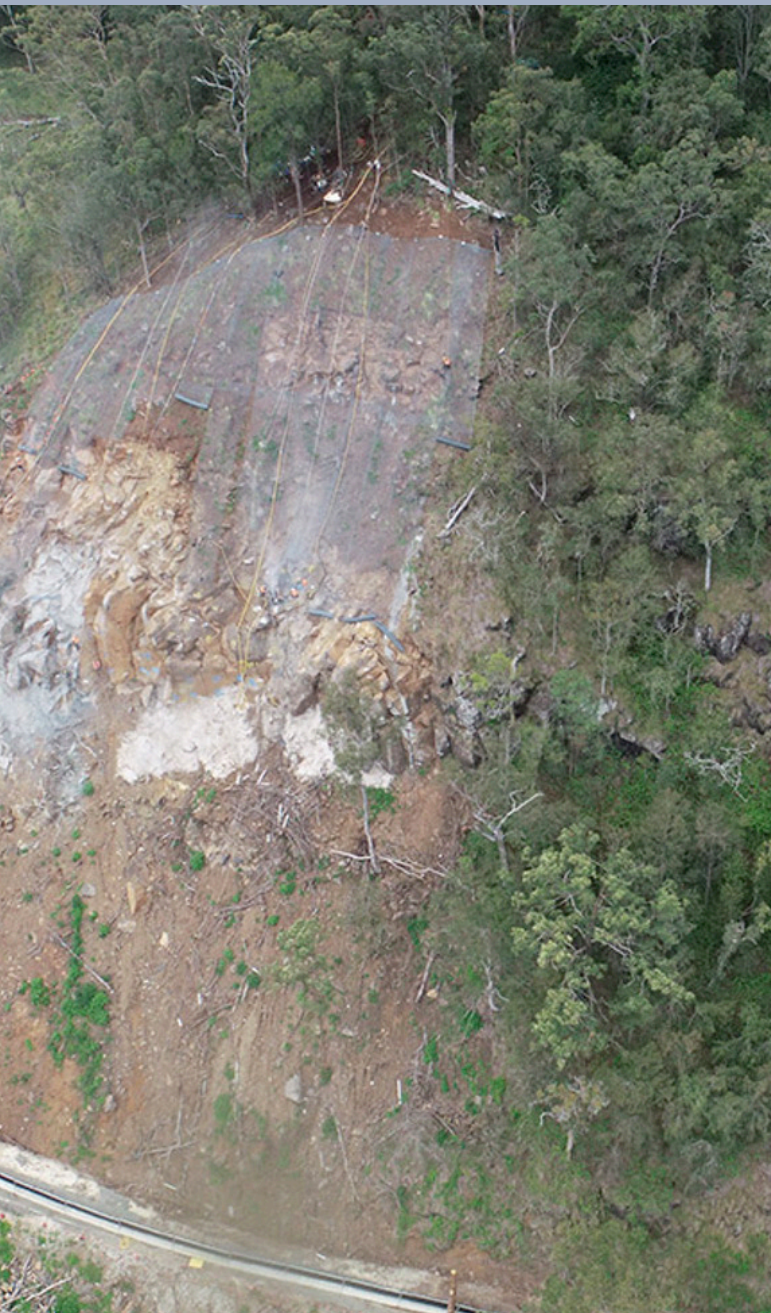
Image: Tamborine Mountain Road – mesh works in progress.
