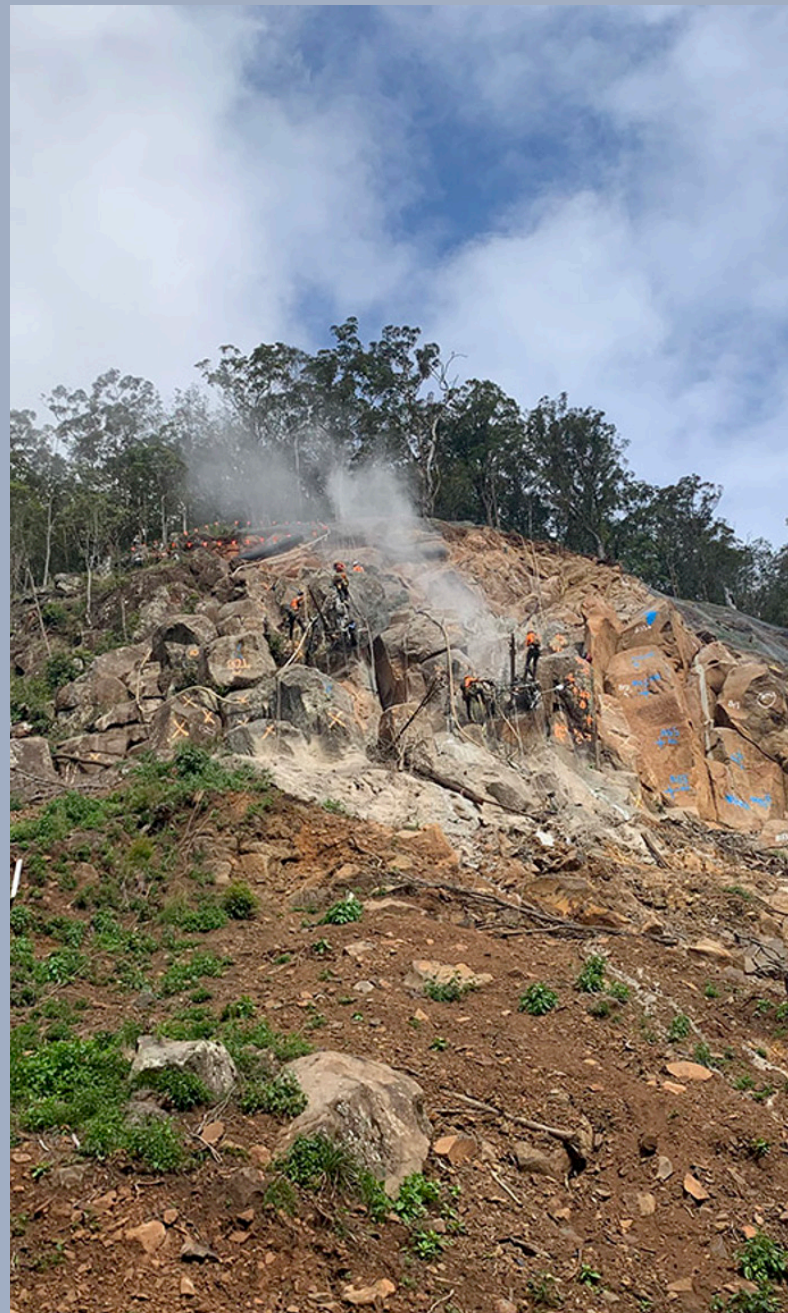
Image: Tamborine Mountain Road – mesh works in progress.
