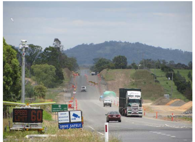
Monitoring equipment on the Cunningham Highway just south of Warwick (near Lyndhurst Lane) – travelling south, this was the first of up to nine sites a motorist would pass through
