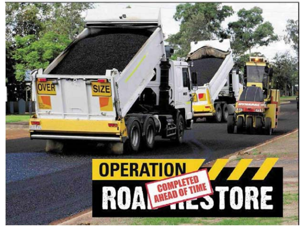
Alice Street in Dalby was a hive of activity as the final works were completed on Council's Operation Road Restore program
