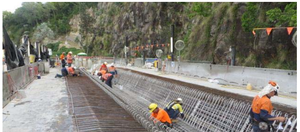
Right: Work on the reinforcement for the girders
