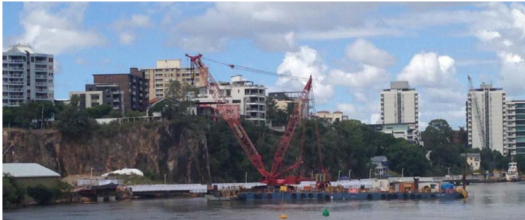
Above: Riverwalk is now taking place with seven girders installed
