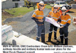
MEN AT WORK: CMC Contractors (from left) William Jackson, Anthony Neville and Anthony Kumar look over plans for the West Creek Channel project. PHOTO: KEVIN FARMER
