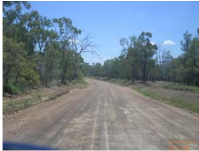
Damage to (top and centre) and following reconstruction works (bottom) to sections of Bluff Jellinbah Road
