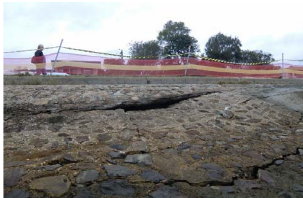
Left: damage to Bongaree Seawall, Bribie Island following storm surges associated with January 2013 disaster event
