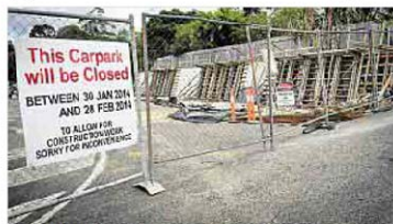
FLOOD REPAIR: Young St car park construction. PHOTO: PATRICK WOODS
