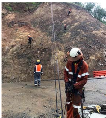
Disaster reconstruction works underway by TMR during November 2017 following impacts of STC Debbie: (left) Lamington National Park Road landslide works; (middle) Soil nailing on upper slope on the Sarina Range; (right) Early works at landslide site on the Sarina Range
