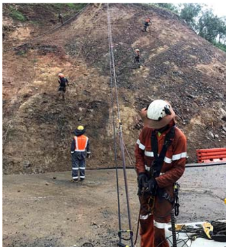
Soil nailing on upper slope at Sarina Range (left)
