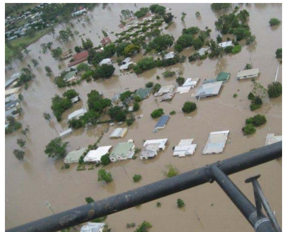
Above: Aerial photo of Mundubbera following Tropical Cyclone Oswald
