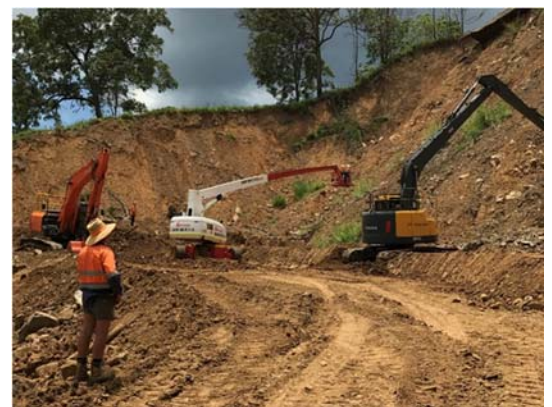
Disaster reconstruction works underway by TMR during November 2017 following impacts of STC Debbie: (left) Lamington National Park Road landslide works; (middle) Soil nailing on upper slope on the Sarina Range; (right) Early works at landslide site on the Sarina Range
