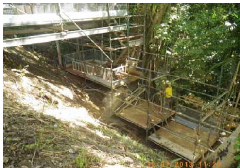
Above: slope stabilisation works below road, Kuranda Range
