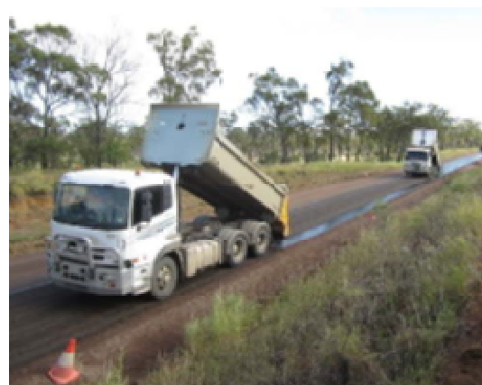
Above: Mackay/Whitsunday Region's Collinsville-Elphinstone Road (West package) – sealing works in Glenden
