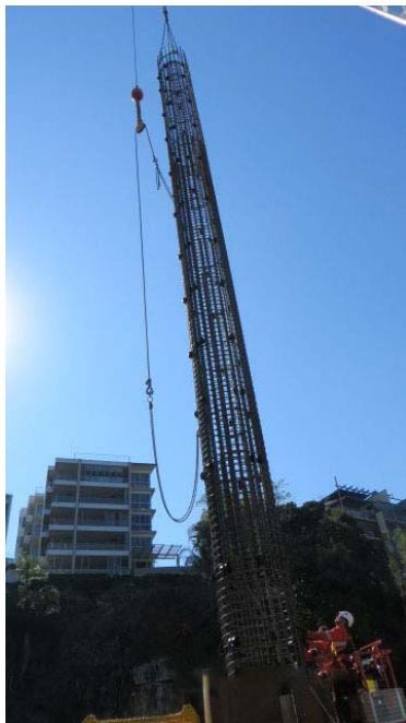
Left: steel reinforcement for a pile is craned into place.
