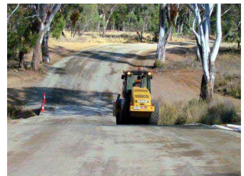
Above: Roma-Taroom Road - rolling off road base
