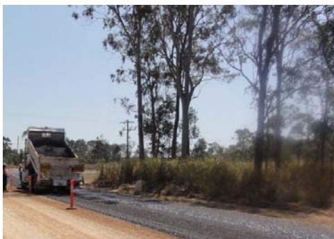
Left: Reconstruction works underway on Awoonga Dam Road
