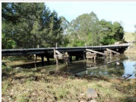
Above: Original Grigor Bridge at Conondale
