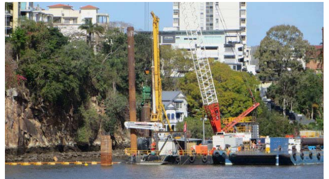
Right and below right: Piling works underway.
