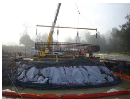
Above: Lifting the cage onto the new bridge pier
