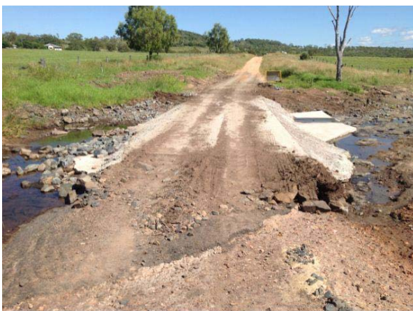
Above: Damage to sections of Mondure-Wheatlands Road (South Burnett Regional Council)
