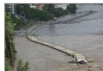
Above: damage to Brisbane RiverWalk during January 2011 floods.
