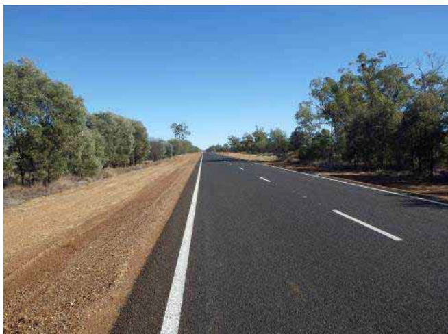
Above: construction works completed—Landsborough Highway (Morven to Augathella)
