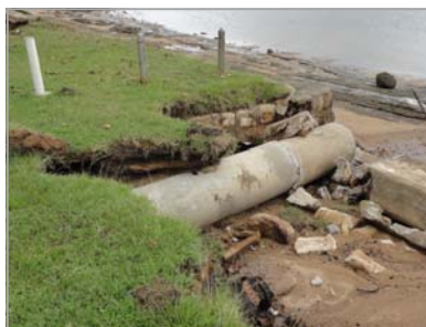
Images above showing damage to sections of Palm Island the seawall following Tropical Cyclone Yasi.
