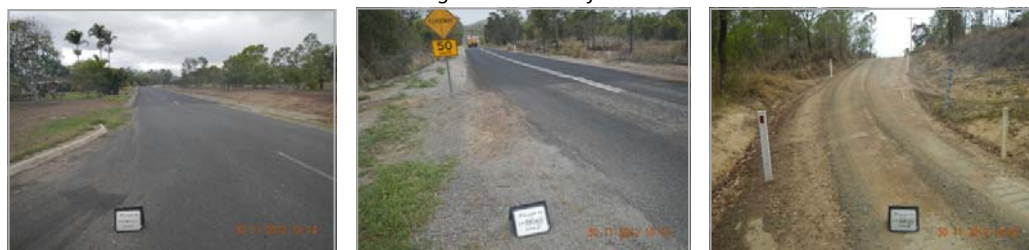
Above: completed works on sections of Bilwon Road.
