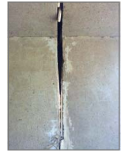
Above: damage from 2013 flooding of culverts on Callandoon Road.
