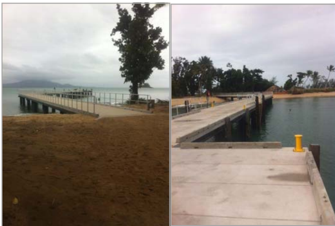
Above: Completed works—Dunk Island jetty.
