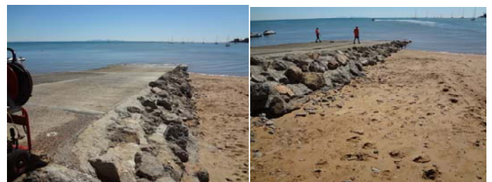
Above: Completed works at Horseshoe Bay boat ramp, Magnetic Island.
