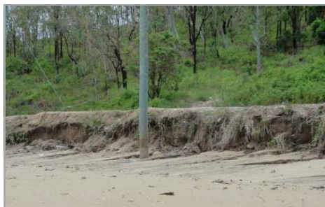
Images above showing damage to sections of Palm Island the seawall following Tropical Cyclone Yasi.
