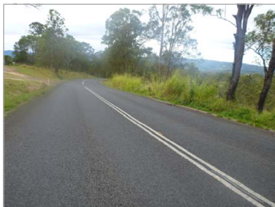
Right: Completed works on a section of Traveston Road.
