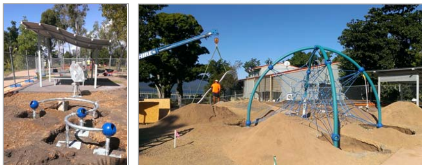
Left : Installation of play equipment on Cardwell Foreshore, June 2013.
