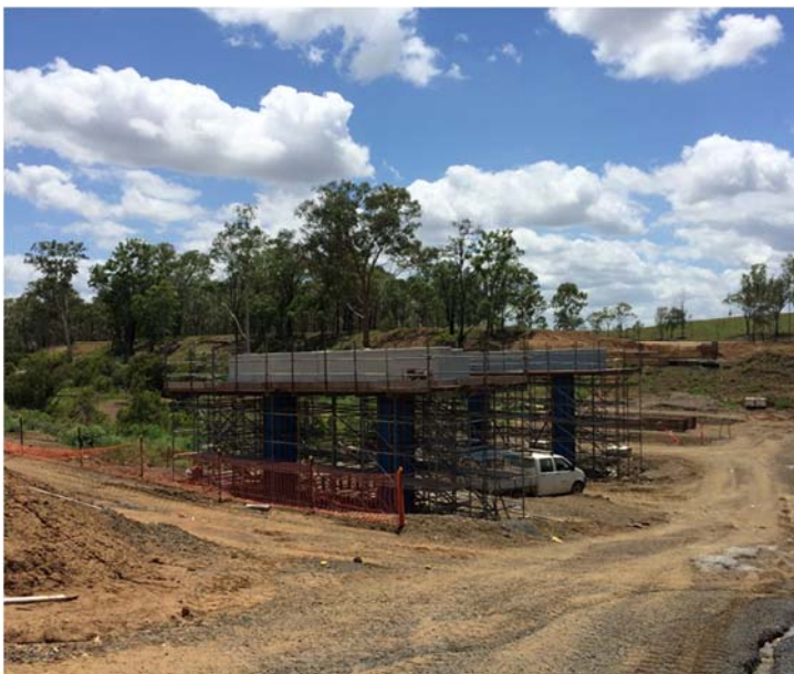
Above: Burnett River Bridge – bridge sub-structure (columns and headstocks)
