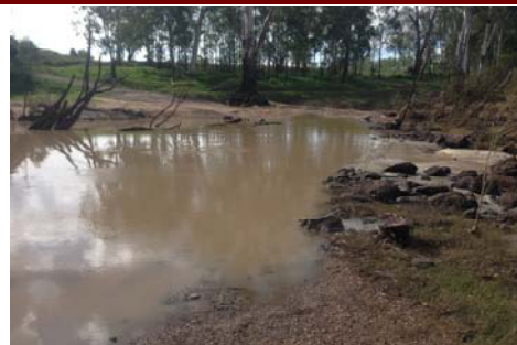
The flooded Aroona Road crossing in 2013
