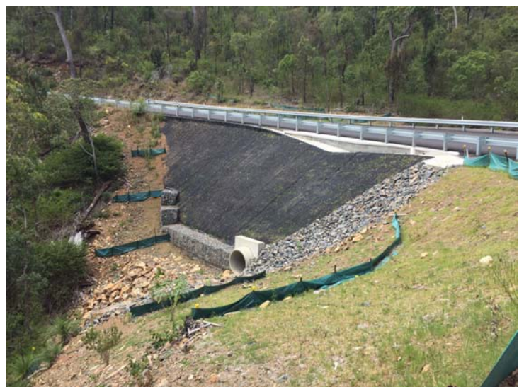
Above: Rockhampton Regional Council's Pilbeam Drive Betterment project during repair and upgrade works and at completion
