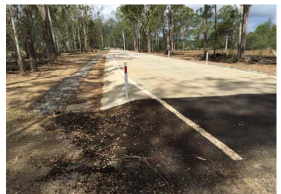
Above: Emerys Bridge Road before and after
