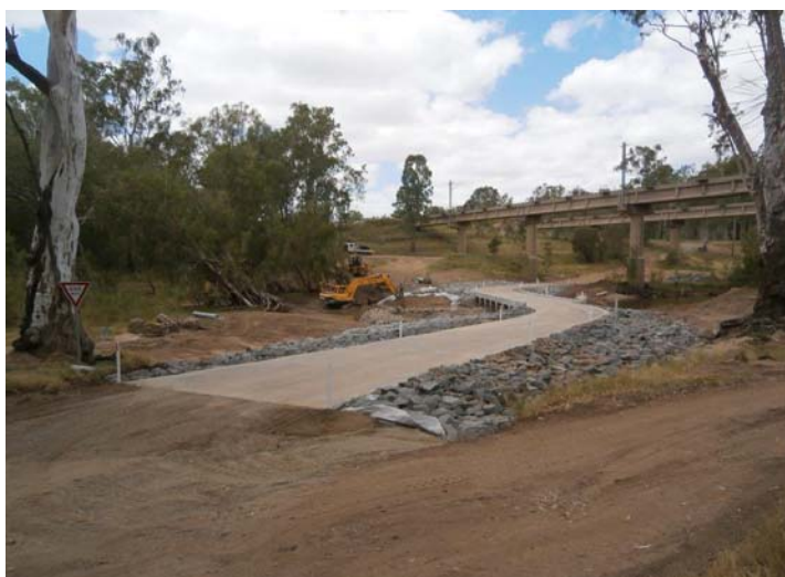
The new resilient Aroona Road crossing – February 2017
