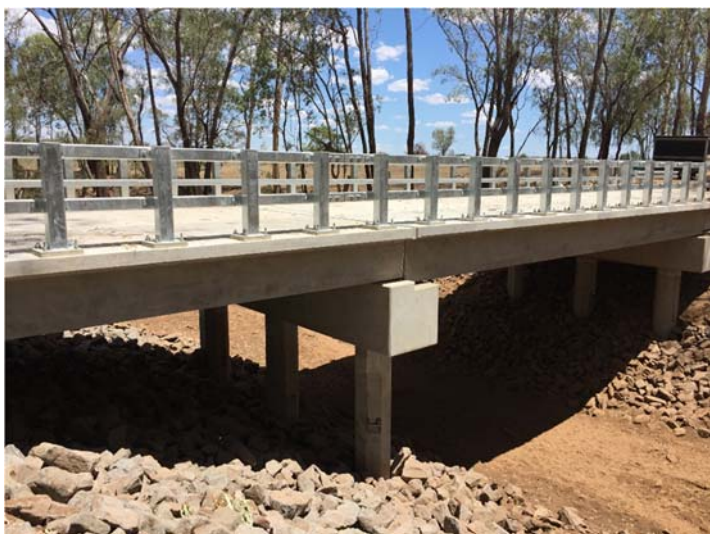
The new and upgraded Herbert Creek Bridge – December 2016
