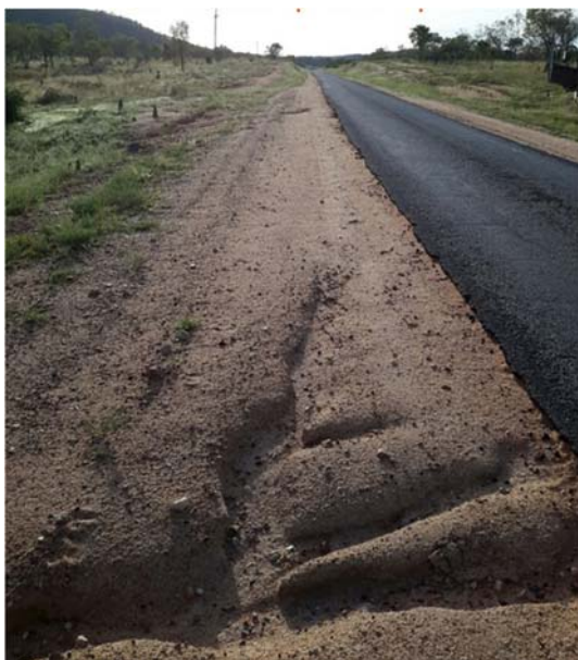
Gulf Developmental Road (Georgetown–Mt Garnet) – damage from Gulf of Carpentaria Monsoon Trough (December 2015–January 2016) (left); and following completion of restoration by TMR (right)
