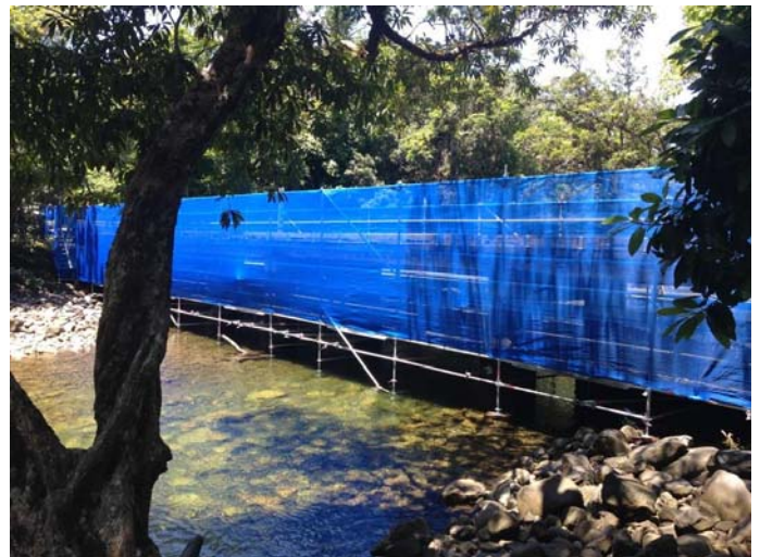
During repairs to Noah's Creek Bridge, temporary scaffolding was erected to protect the World Heritage listed Daintree Rainforest.
