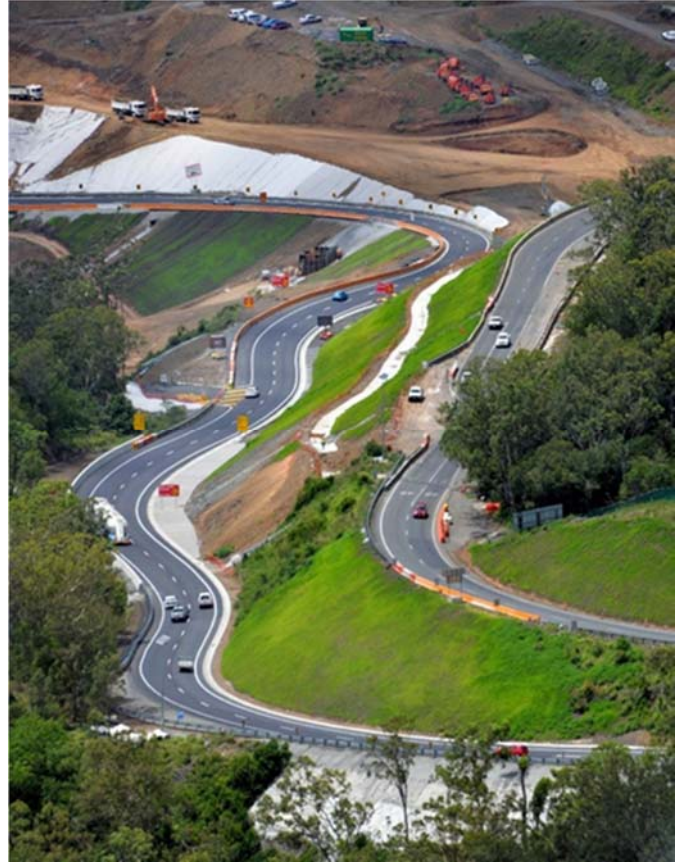
Completed works on Toowoomba Range – eastbound section
