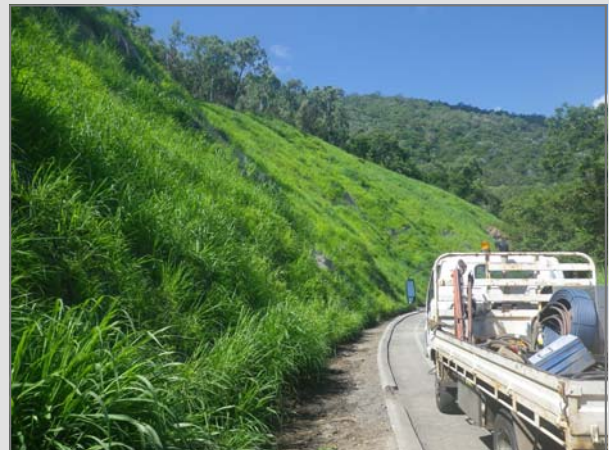
Above: Slope stabilisation works completed
