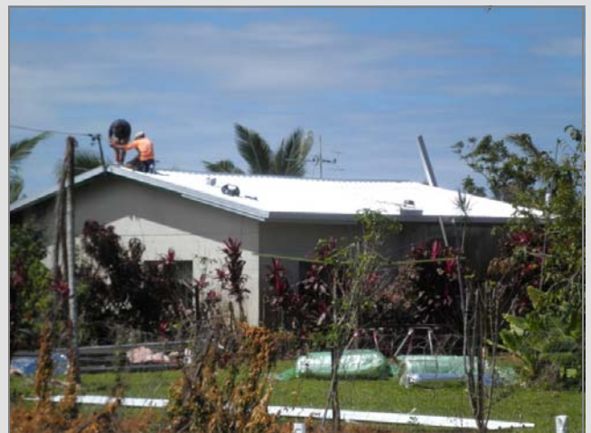
Above: Mr Vidmar's home being repaired
