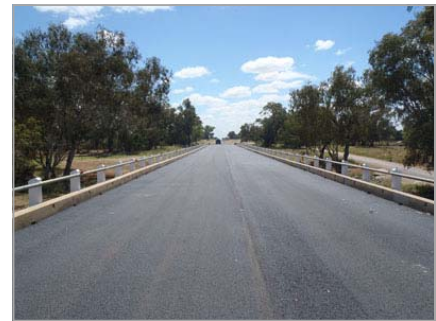
Above: Completed bridge now open to traffic.
