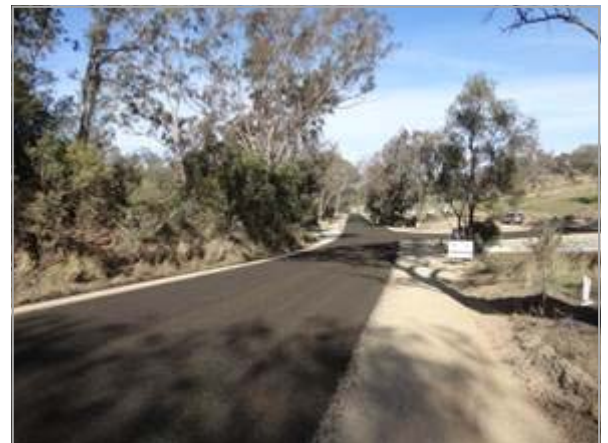
Above: Gowrie-Glencoe Road following reconstruction.
