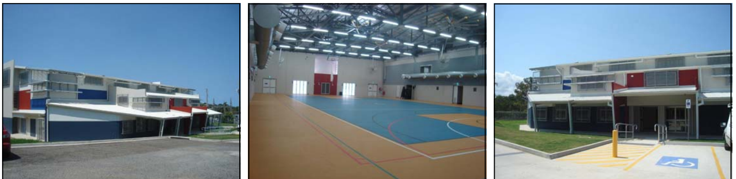
Above: Cyclone Shelter - Yeppoon SHS - officially opened on 14 November 2012.
