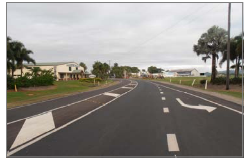
Above: Completed section of Bruce Highway.
