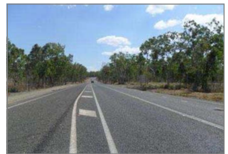
Above: Peak Downs Highway – completed section.
