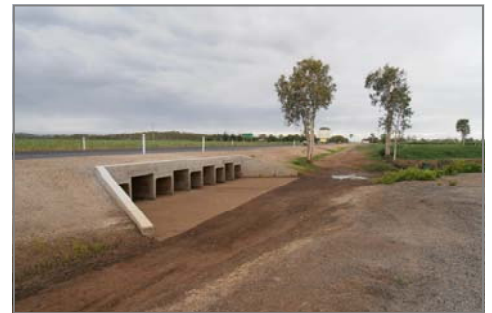
Above: Completed section of Bruce Highway
