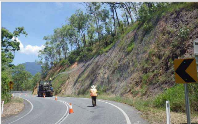
Above: Gillies Range Road—slope stabilisation works in progress
