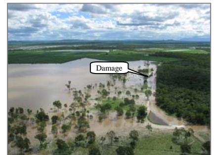
Above: Aerial view of flooded Groper Creek Road showing a damaged section.
