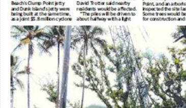
DRIVING FORCE: Construction work on a jetty at Clump Pt.
