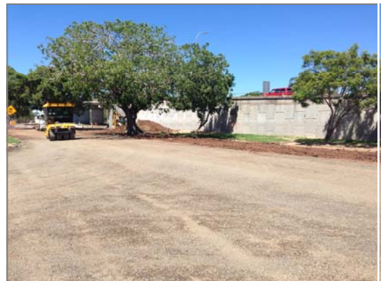
Above: Don Tallon Bridge after the completion of emergent works
