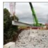
Right: concrete span being shifted into place
