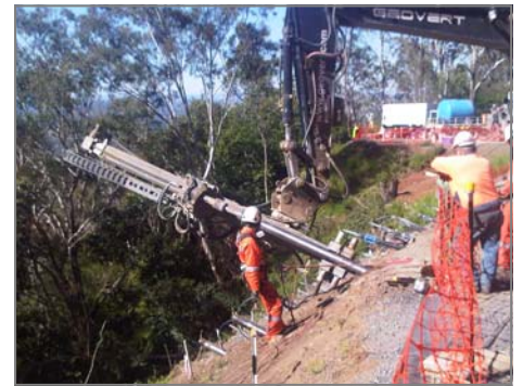
Above: Soil-nailing underway to repair a section of the Toowoomba Range
