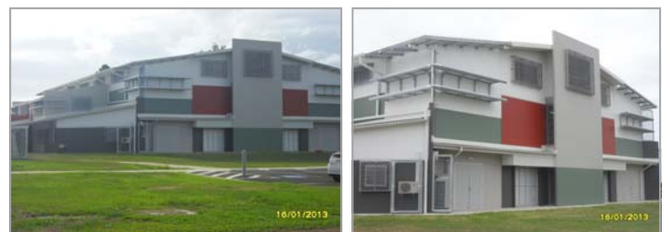
Above: Recent photos of the completed Ingham Cyclone Shelter - with greener pastures
