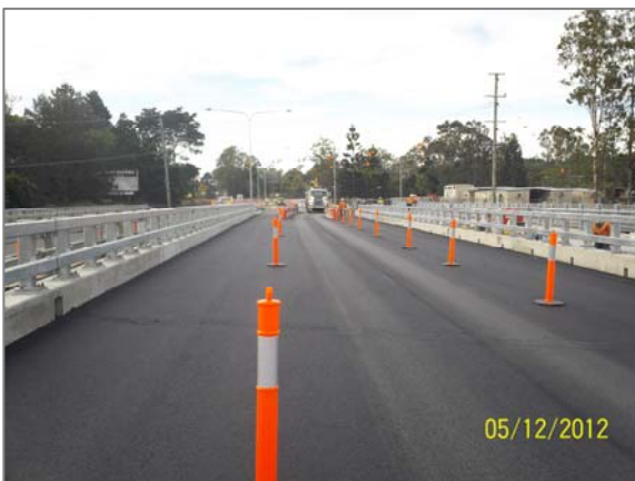
Above: AJ Wyllie Northbound Bridge prior to reopening celebration.
