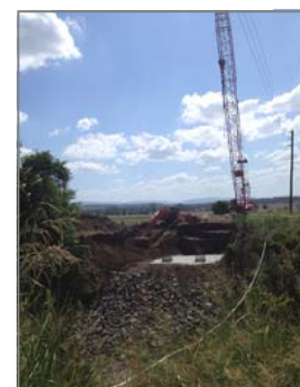
Above: construction of headwall and piles at abutments.
