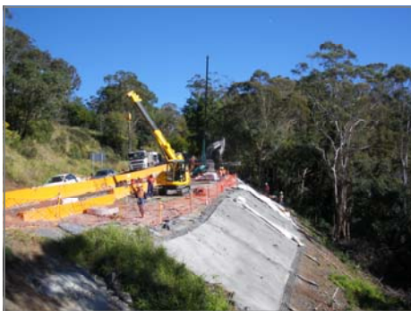
Above: Slope stabilisation works on a section of the Toowoomba Range crossing, Warrego Highway
