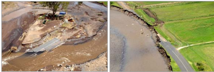
Above: Damage to sections of Mt Sylvania Road following the 2013 event
