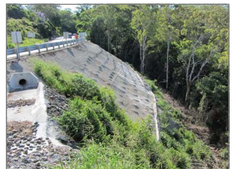
Above: Completed works on a section of the Toowoomba Range crossing
