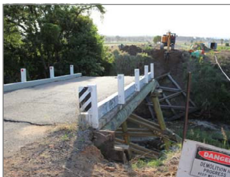
Above: removal of the damaged bridge
